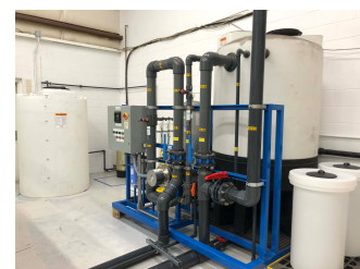
Process Solutions' in-house membrane cleaning plant is up and running!
