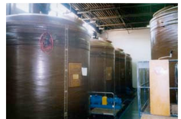
Fiberglass storage tanks
