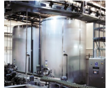
Stainless steel storage tanks
